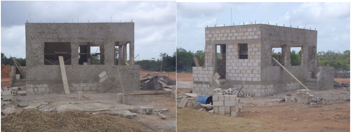
Administration Building Construction Progress
