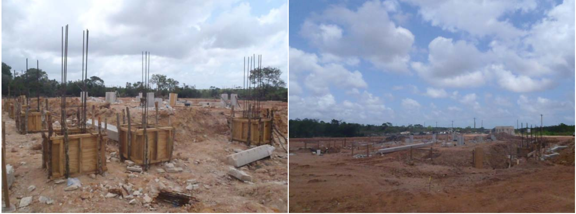
Transfer Station pile in place
